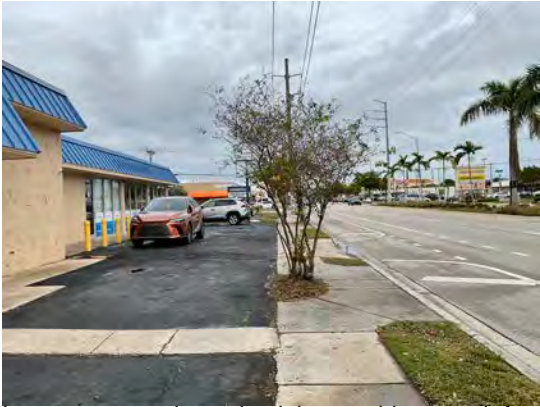
In many areas, the setback is not wide enough for parking, is impervious and lack a buffer to sidewalk.
