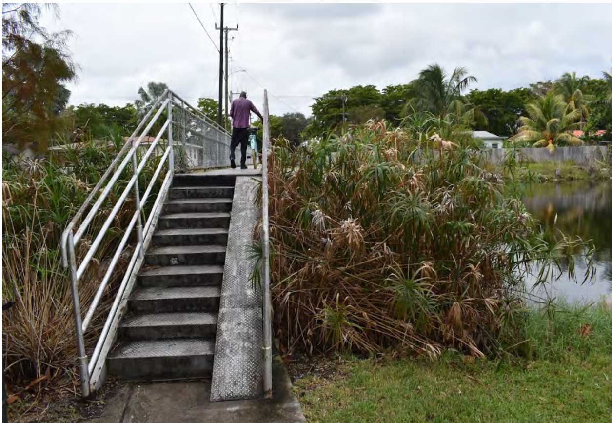
A future bridge will be wider to accommodate pedestrians and bikes and be universally accessible.
