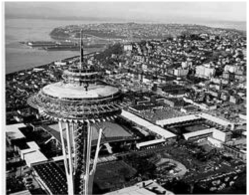
Space Needle and Seattle Center under construction.
