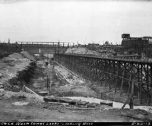
Hiram M. Chittenden Locks under construction.
